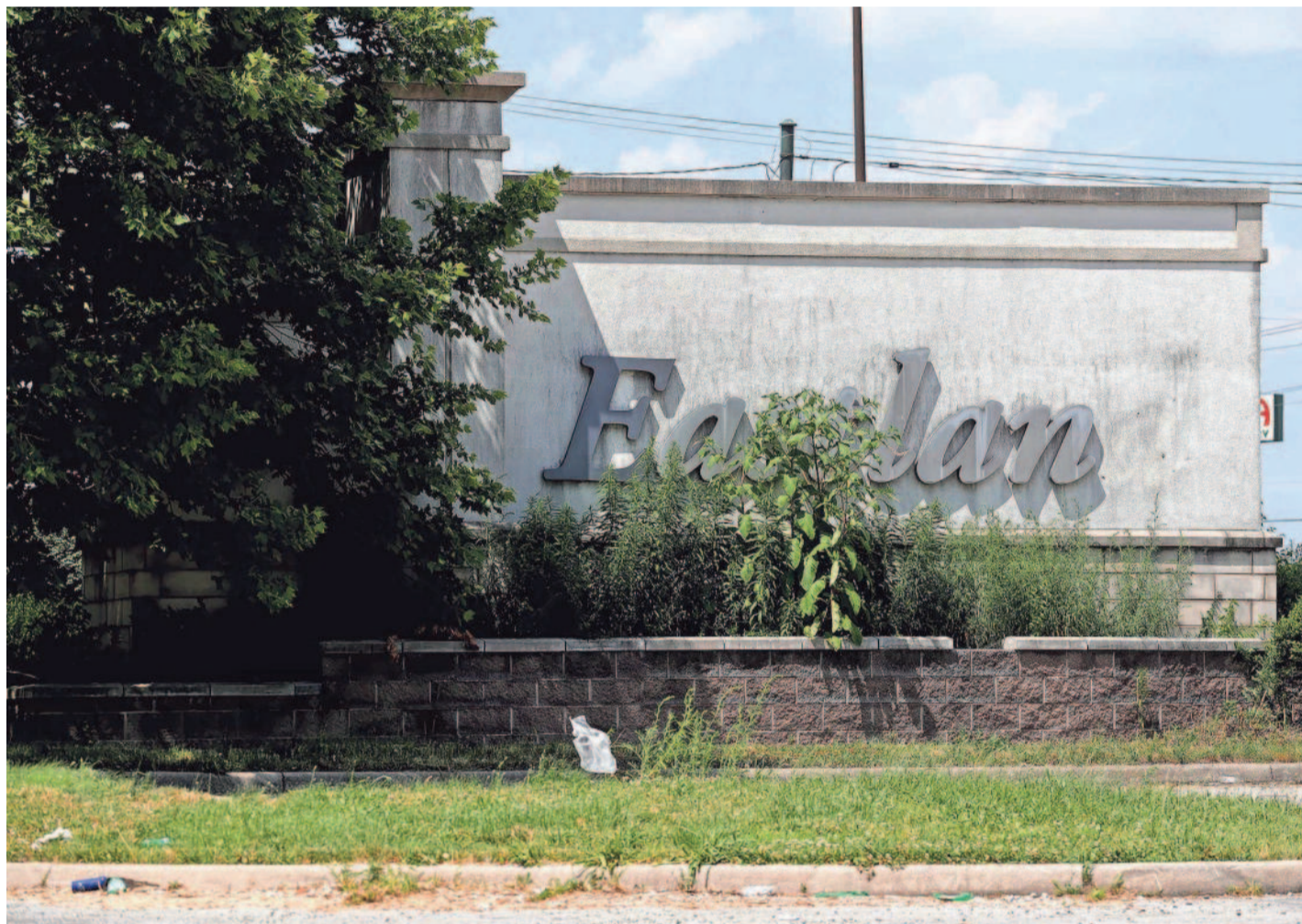
Trash, weeds and a missing “d” greet visitors who enter one of Eastland Mall’s parking lot entrances. A Columbus judge is requiring the owners of the mall to make repairs and improvements or else the city could take control of the mall or even demolish it. Meanwhile, the owners of many of the mall’s businesses say they’re struggling.
